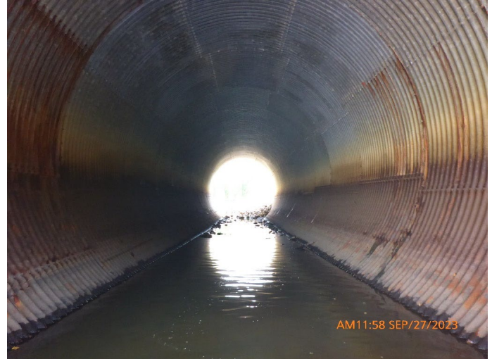
Figure 68 Fair Condition Culvert Example
