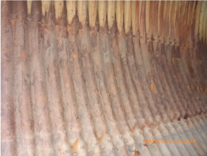
Figure 68 Fair Condition Culvert Example
