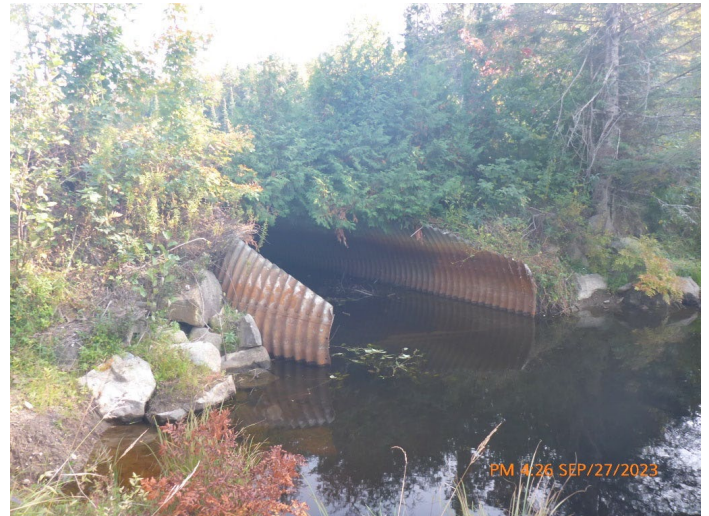
Figure 69 Poor Condition Culvert Example
