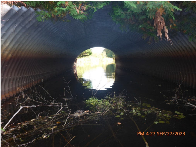
Figure 69 Poor Condition Culvert Example
