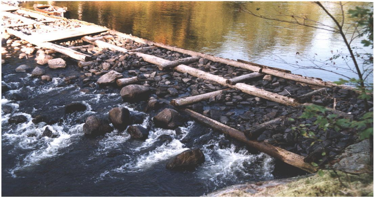
Figure 1 – The Previous Rock and Crib Dam (September 1998)
