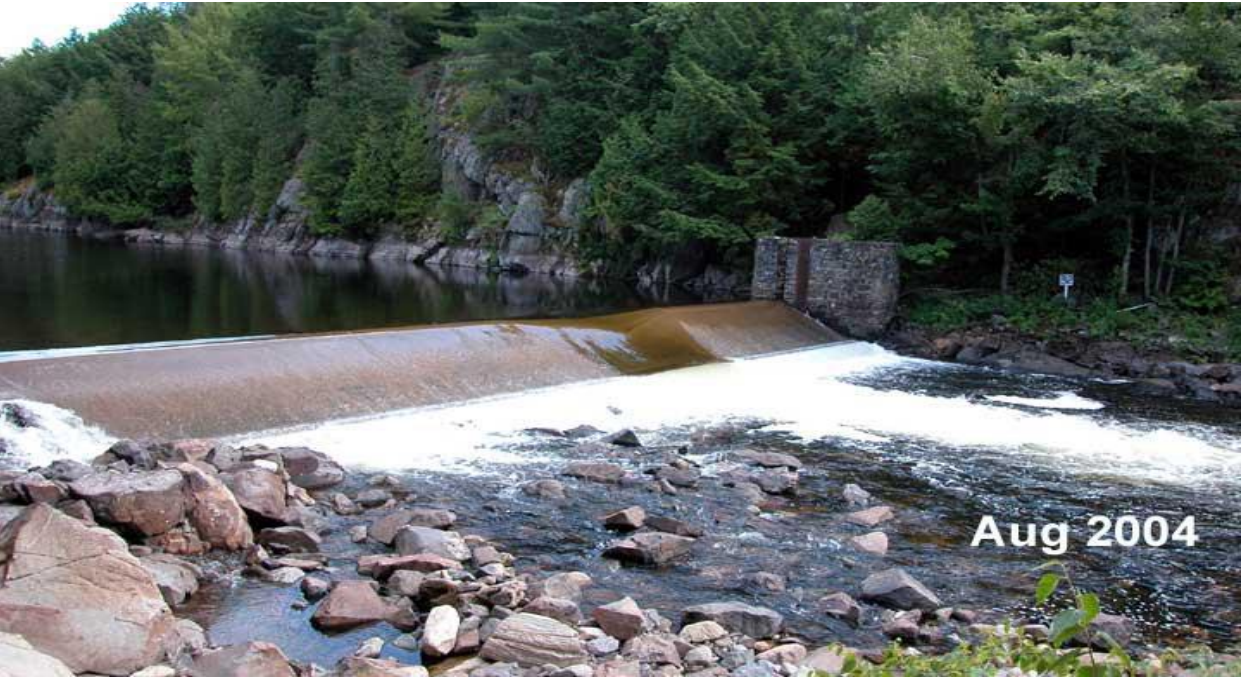
Figure 2 – Current Dam after Completion in August, 2002
